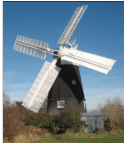
Wicken Mill, Cambs, received a grant from the Mills Repair Fund.
