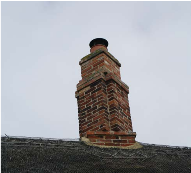
Figure 31: Chimney height raised on thatched cottage. Photo: © Douglas D Kent
