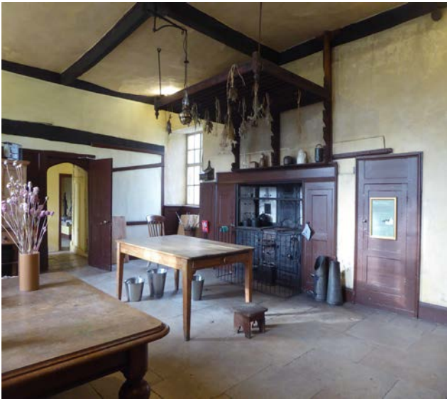
Figure 6: Kitchen, c1300-1900s. Manor Farm, Cogges, Oxfordshire. Open hall with inserted floor, lateral chimney stack with wide fireplace, later inserted cooking range and side cupboards. Note the spit rack above the fireplace. Photo: © Heather Horner, with thanks to Cogges Heritage Trust
