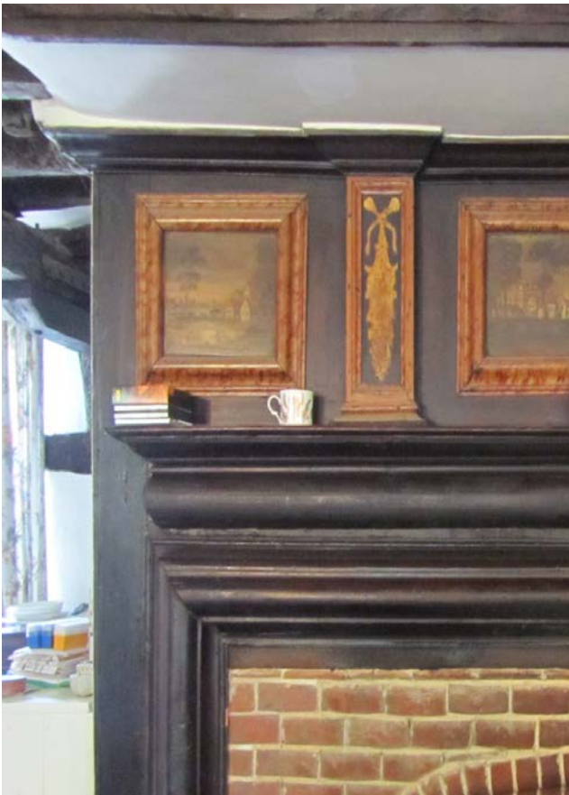
Figure 10: Detail, fireplace with bolection moulding, c1700s. Steventon, Oxfordshire. Photo: Sally Stradling
