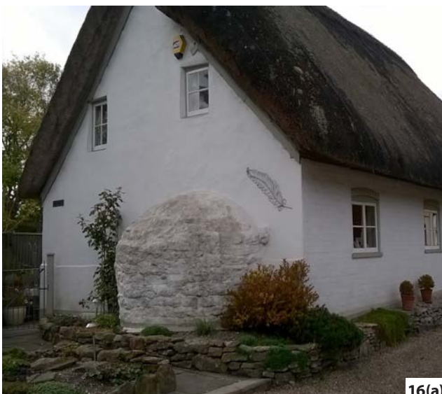
Figure 16: Bread ovens: (a) Bread oven 'bulge'. East Hanney, Oxfordshire. (b) Interior of bread oven showing brick lining. Old Priest's House, West Hoathly, West Sussex Photos: Sally Stradling (a) and Matthew Slocombe (b)
