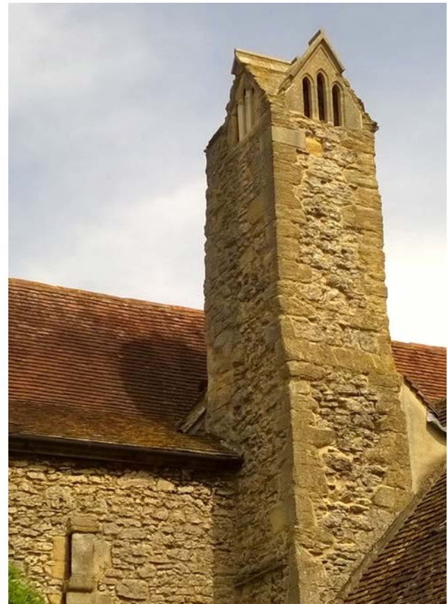
Figure 4: Flue with triplets of lancets, c1260. The Checker, Abingdon Abbey,
