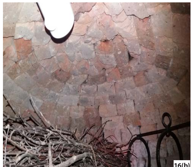
Figure 16: Bread ovens: (a) Bread oven 'bulge'. East Hanney, Oxfordshire. (b) Interior of bread oven showing brick lining. Old Priest's House, West Hoathly, West Sussex Photos: Sally Stradling (a) and Matthew Slocombe (b)
