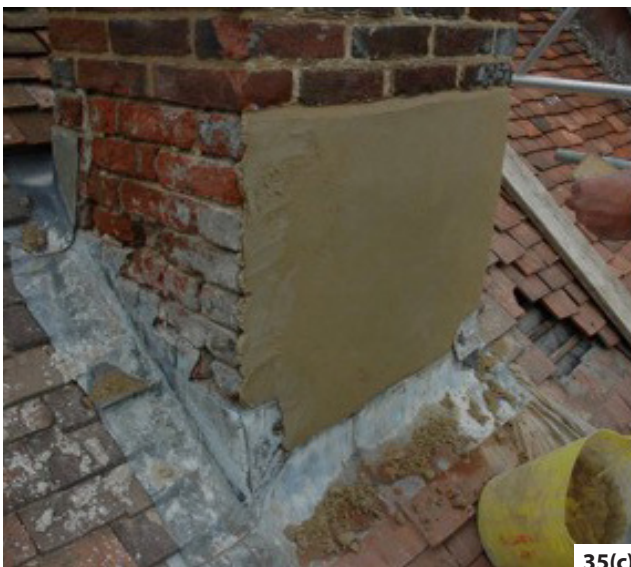
Figure 35: The repair of a damp chimney stack that had been coated in cement render: (a) After removing the render, new lead 'soakers' were inserted to prevent rain entering at the junction between roof and stack. (b) A continuous lead flashing was fixed to the brickwork, set into the lime mortar joints. (c) Finally the damaged brick was rendered with a lime mix. Photo: Marianne Sühr
