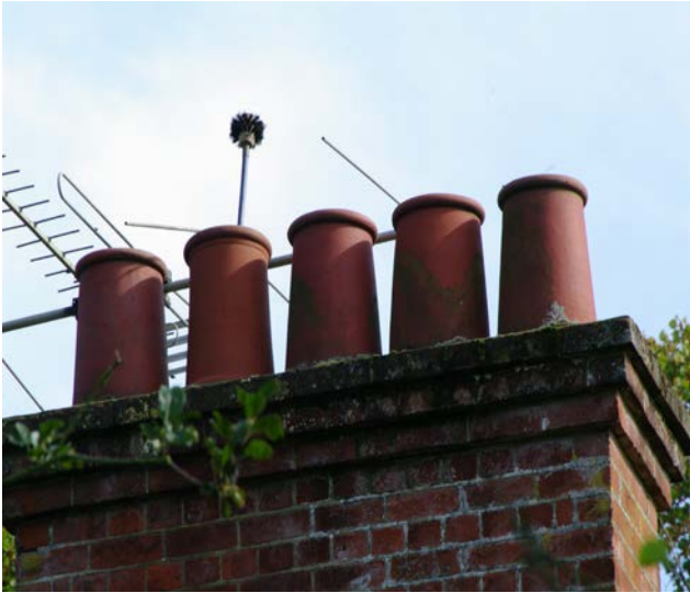
Figure 30: Chimney sweeping. Photo: © Douglas D Kent
