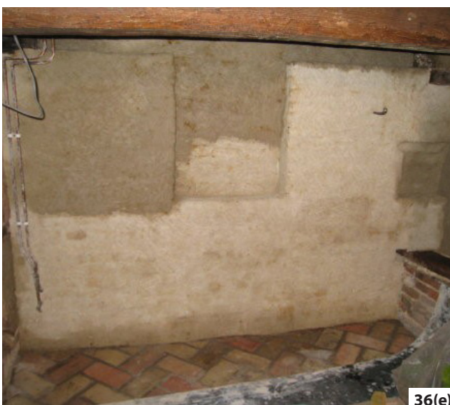
Figure 36: Using cow dung to prevent tar leaching in old chimneys: (a) Tar on bricks. (b) Two coats of fresh cow dung diluted to the consistency of ice cream are brushed on first, allowing thorough drying between them. (c) Manure is mixed into a scratch coat in a ratio of 3:9:1 lime: sand: manure. (d) The surface is worked, any cracks trowelled up with a wooden float as they appear and a key scratched when the coat is green hard. (e) A second lime coat and lime skin are applied as normal. (f) Finished inglenook with breathable paint. Photos: © Yvonne Reynoldson
