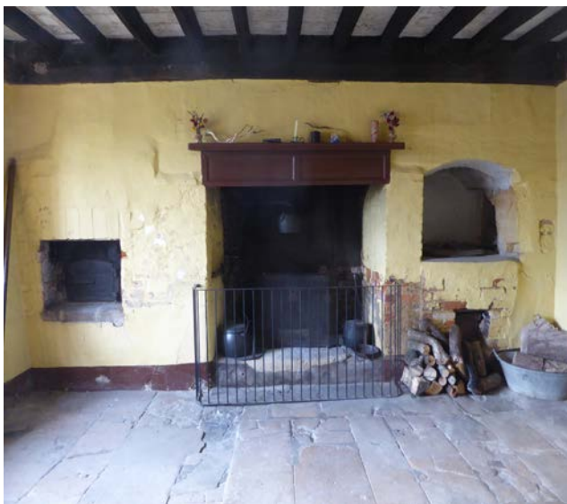
Figure 8: 'Back kitchen', c1600s-1900s. Manor Farm, Cogges, Oxfordshire. Main range in centre, bread oven to left, copper for washing clothes to right. Photo: © Heather Horner, with thanks to Cogges Heritage Trust
