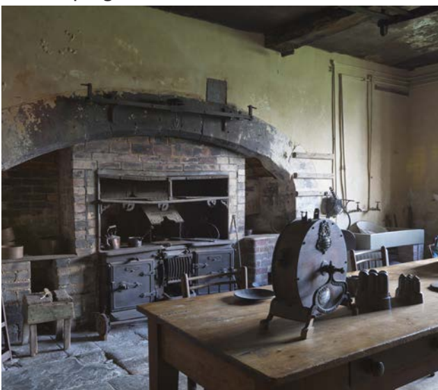
Figure 5: Kitchen fireplace c1600s. Chastleton House, Oxfordshire. Note the width of the fireplace and insertion of later cast iron range and copper.
