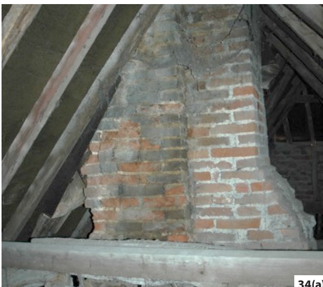
Figure 34: A 17th-century stack viewed from the roof space (a). Note the erosion of the brickwork just below the roofline, causing the stack to become structurally unstable. (b) The same stack was repaired by a highly skilled bricklayer who propped it, opened up the roof and replaced the damaged bricks one by one. Photo: Marianne Sühr
