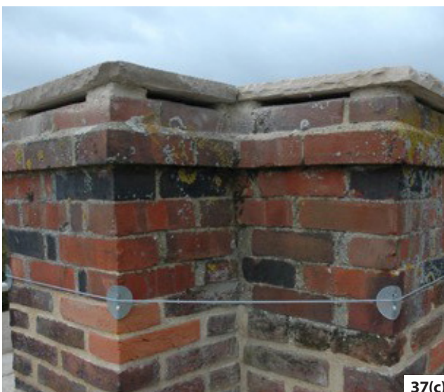
Figure 37: Chimney termination: (a) The stack shown in figure 34 from above. Note the exposure to the weather and previous attempts at repair using cement-based mortars. (b) The top of the stack protected with new stone slabs. The two redundant flues have complete slabs, the working flue has a stone capping to the brickwork. (c) The redundant flues have air slots to prevent condensation. (d) The finished stack, repaired using hydraulic lime mortar.
