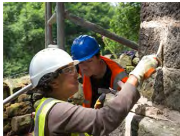
RIGHT BELOW → Repointing at the Lumsdale Working Party CREDIT: RALPH HODGSON
