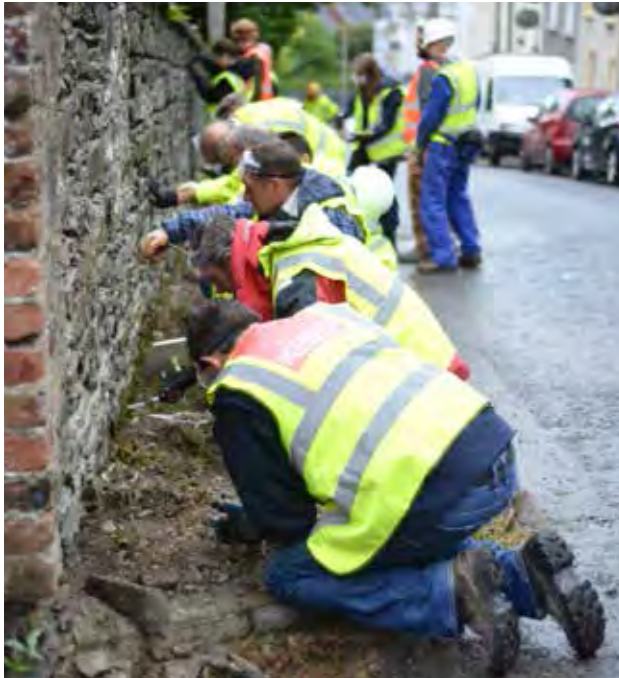
ABOVE Hands-on conservation with SPAB Ireland: teaching volunteers to prepare and work with hot-mixed lime mortars. CREDIT: JOHN MCDAID
